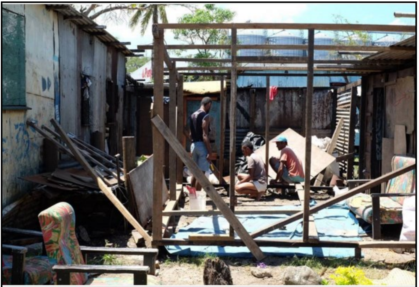
Three men investigating the destruction of houses in the wake of TC Winston © IOM 2016 (Photo: Joe Lowry)
